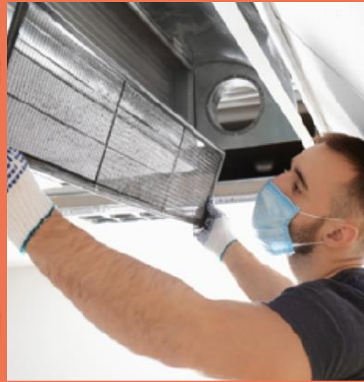
Increased filtration within the HVAC
